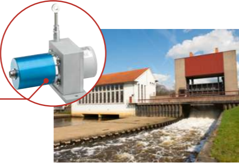
▲ Valve opening control
