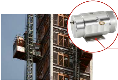
▲ Lift system displacement measurement
